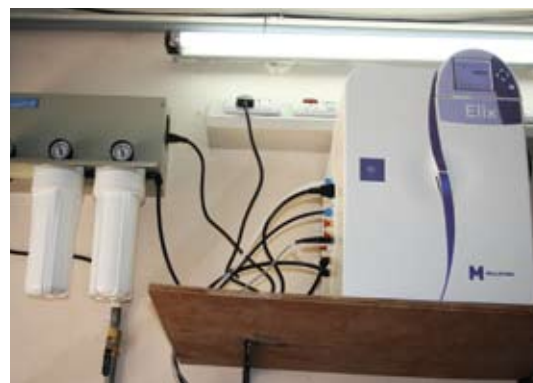
Water Purification System
